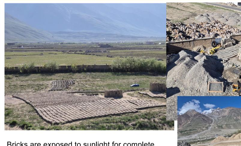
Bricks are exposed to sunlight for complete drying before being laid on the wall. To ensure better bonding and structural strength.
