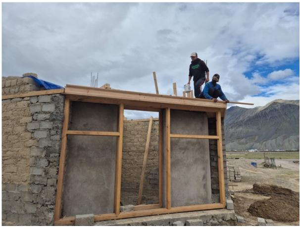
The installation of exterior windows has commenced for the side rooms. Skilled technicians are carrying out the process with precision, ensuring proper alignment and positioning. A water level pipe is employed to verify both horizontal and vertical alignment, thereby guaranteeing accuracy and uniformity across all window Frames.
