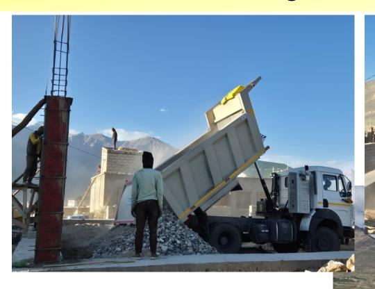
After raising the foundation up to 3 feet above ground level, we have started filling the foundation with gravel of random sizes. The filling is carried out with proper levelling using shovels, and labourers have ensured an even surface. On top of the gravel filling, insulation will be provided using straw-clay bricks, followed by a 4-inch layer of PPC (Portland Pozzolana Cement). Finally, the structure will be completed with finished wooden flooring.
